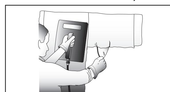
steamed. By working in this way you should be able to remove paper continually. You may have to leave the plate against the wall for longer periods with some papers or re-steam if not completely removed.
