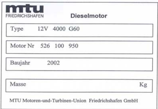
Figure 1.3: Example of generating set identification plate
